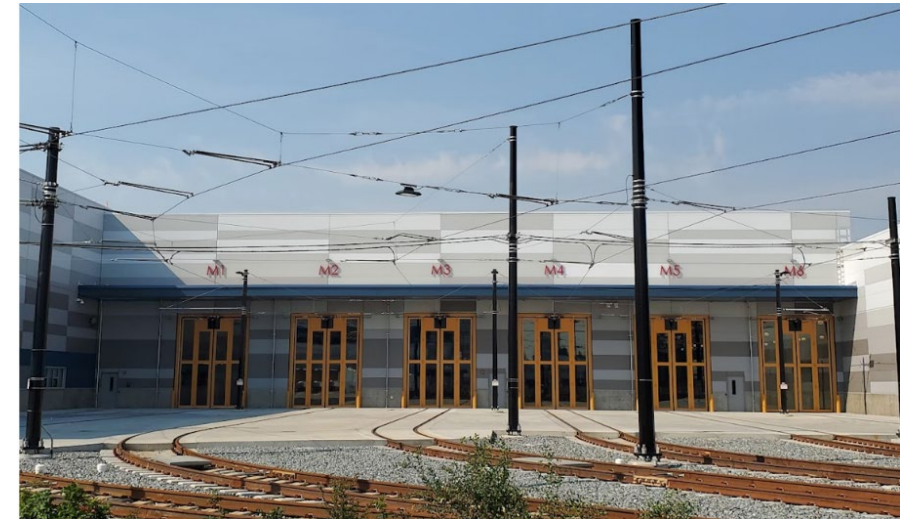
Facility OCS [Source: Mott MacDonald]
