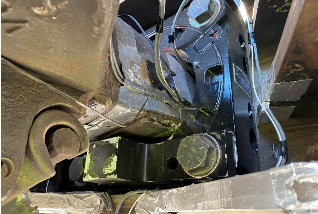
Figure 70. Damage to the limit stop mounted to the front of the sliding lug due to contact by the back of the PBC coupler head
