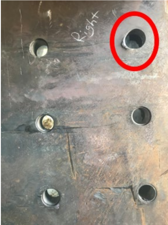
Figure 76. Draft pocket deformed bolt hole
