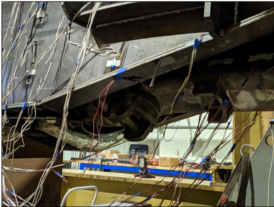
Figure 43. Draft Sill and Bolt Failure – View 2
