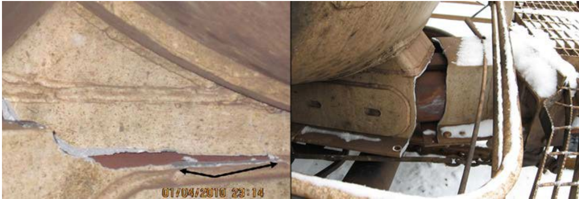
Figure 2. Stub Sill Fracture Observed in Charleston, WV, from January 2010 (Sundaram, 2014)
