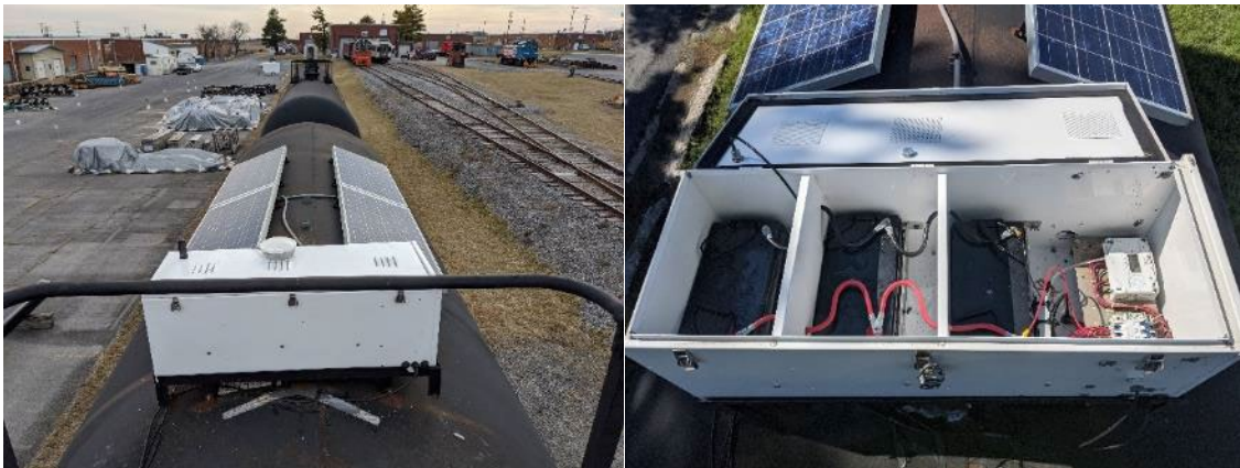
Figure 16. Solar Panel and Battery Box on Top of Instrumented Tank Car
