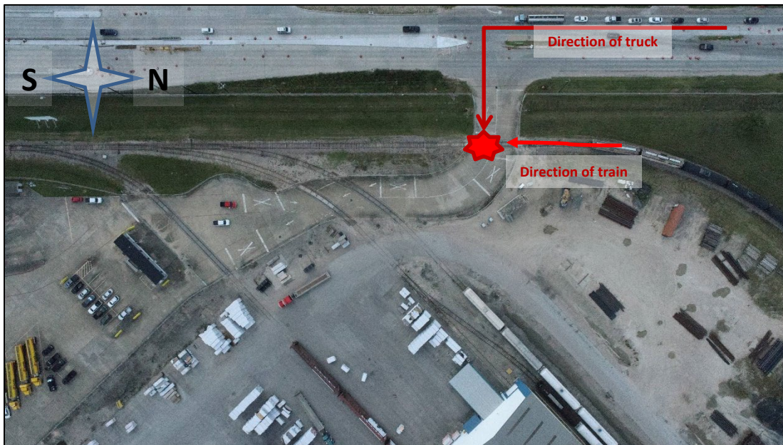
Figure 1: Aerial view of Federal Road and Greens Port Industrial Park
