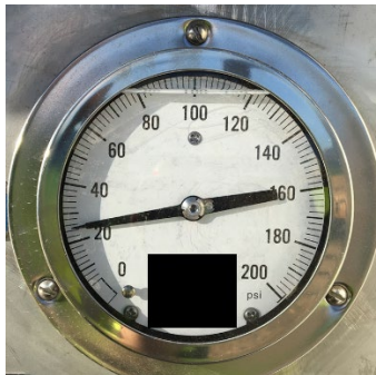
Figure 41. Mechanical Pressure Gauge Prior to Test
