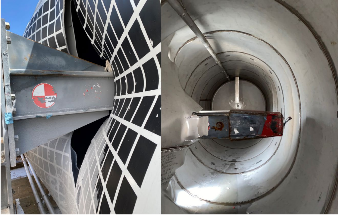
Figure 19. Exterior (left) and Interior (right) Views of Tank Damages from West Side Prior to Impactor Removal
