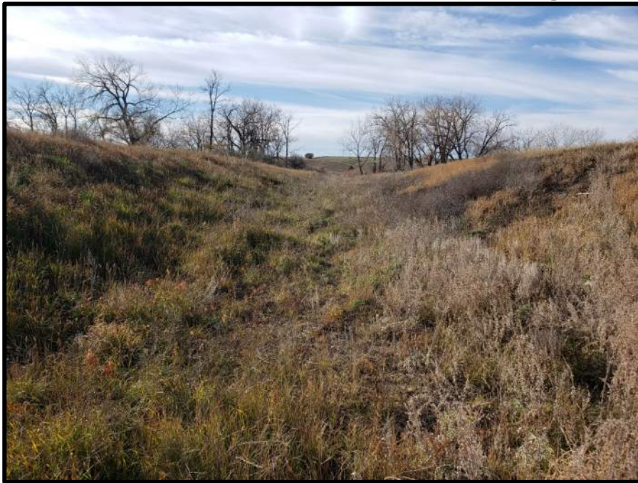
Photo 54. Direction: West. OW8 Stormwater swale.
