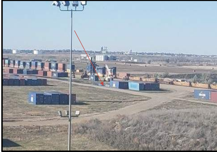
Photo 5. Direction: NW. Wetland 3; standing water near containers.
