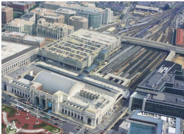
EXISTING STATION CONDITIONS
