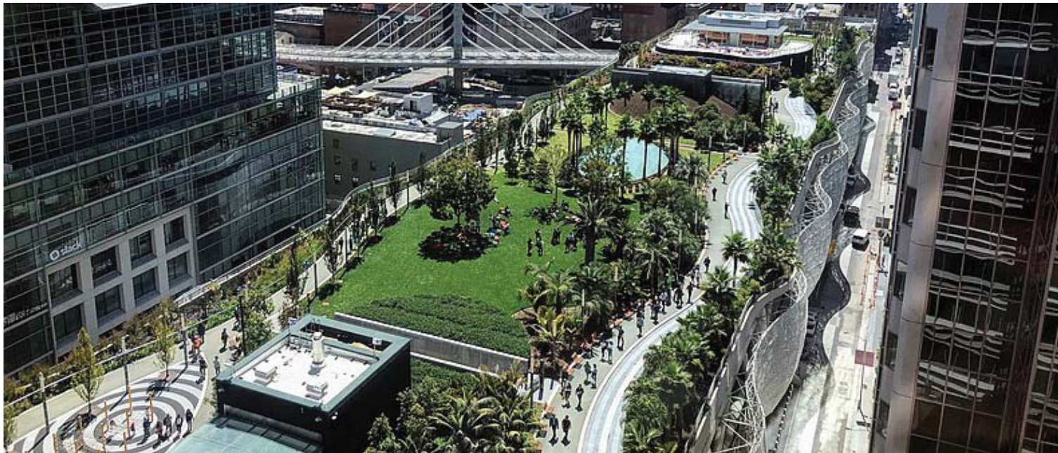
Salesforce Transit Center, Bus Terminal, San Francisco
