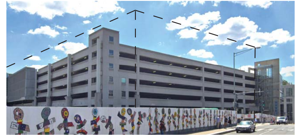
H Street, NE Parking Garage
