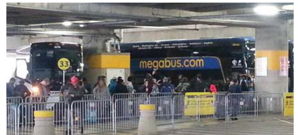
Existing Bus Facility, Union Station
