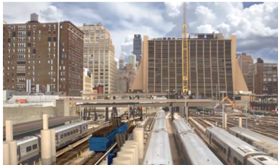
Work trains / Crane location adjacent/above active tracks
