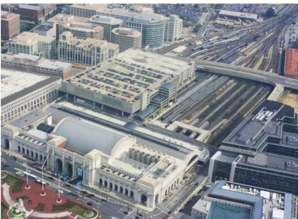
EXISTING STATION CONDITIONS
