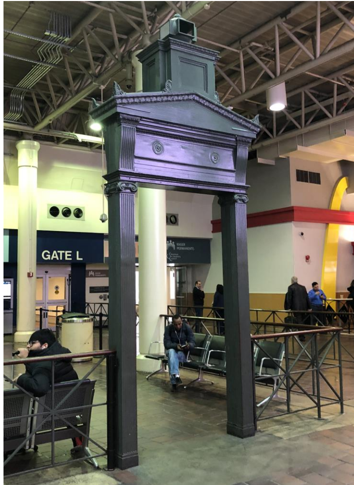
Figure 6. Salvaged gate from the original passenger concourse now serves as a gate to the waiting area in the Claytor Concourse. Source: Dana Litowitz, Beyer Blinder Belle
