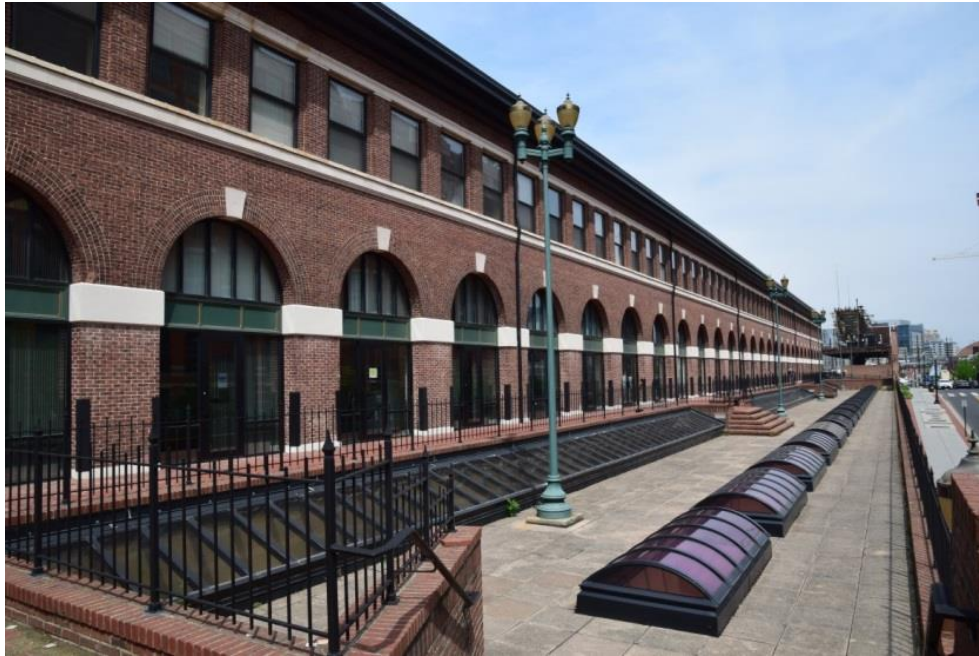
Figure 10. REA Building's east façade, looking northeast. Source: BBB, 2017.
