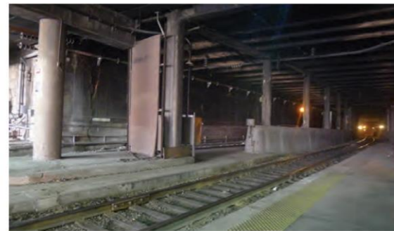
3. North portal of the First Street Tunnel, 2014
