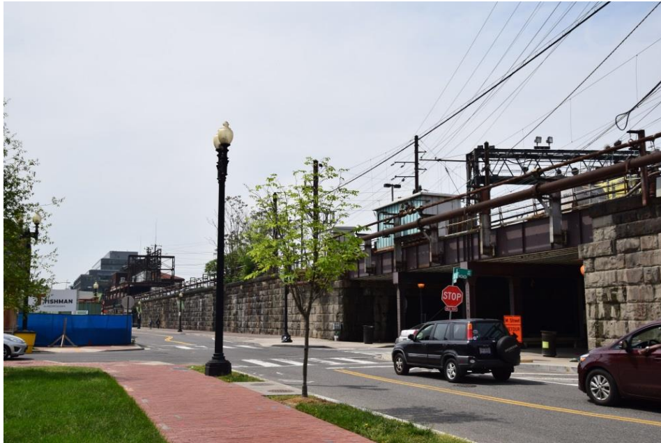
Figure 20. Photograph of L Street underpass and eastern retaining walls, looking southwest. An original signal bridge is visible above the underpass, and Substation 25A is visible on the left. Source: BBB, 2017.
