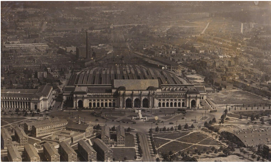
Figure 9. Ca. 1920 aerial view of WUS Historic Site showing south elevation of Union Station, Columbus Plaza, and the expanse of the Terminal Rail Yard to the north. Source: “Lot of Three Post WWI Photos Washington DC Union Station Terminal 1920s,”Ebay, accessed June 21, 2018, https://www.ebay.com/itm/Lot-of-Three-3-Post-WWI-Photos-Washington-DC-Union-Station-Terminal-1920s-/332689707032?oid=332653940455 .
