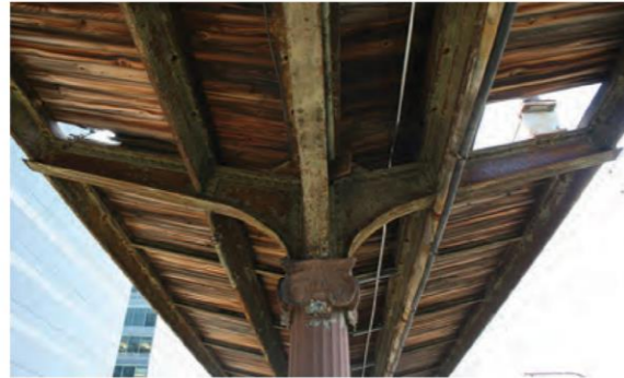
2. Umbrella shed and column capital, 2014
