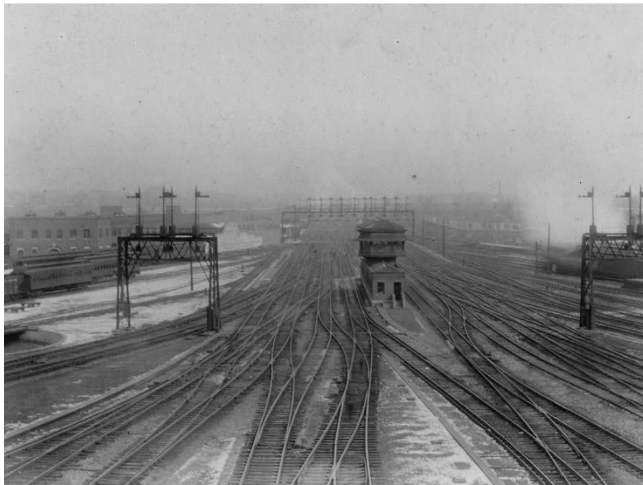
Figure 35. K Tower standing between two signal bridges, looking north, circa 1909. Source: Unknown. Between 1909 and 1932. Photograph. From the Library of Congress, https://www.loc.gov/item/97503313/ .
