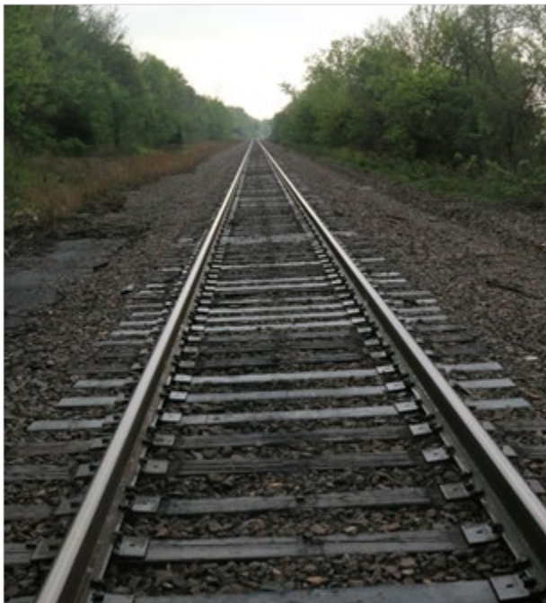
Figure 2. Composite ties inserted one-for-one with wood ties in Chester, Illinois
