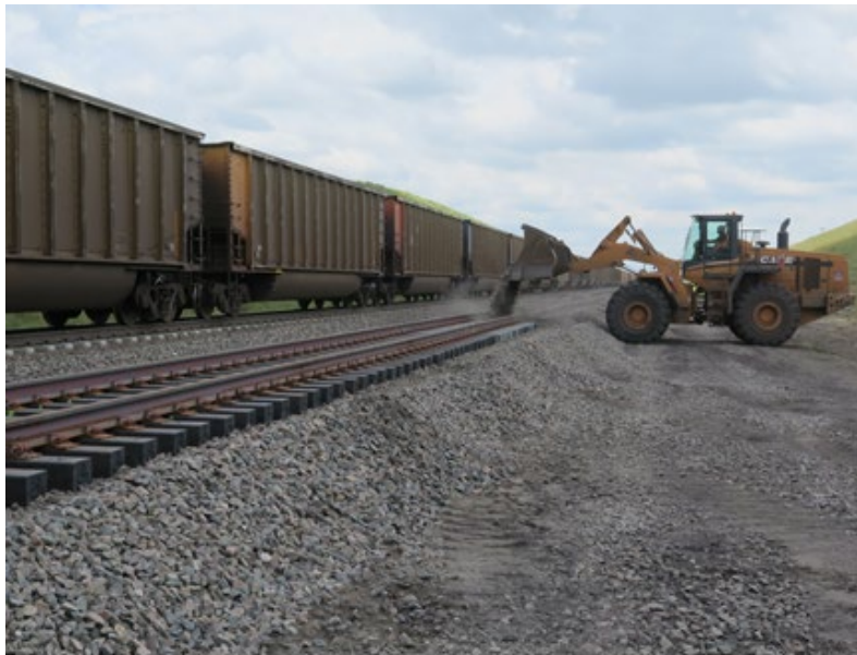
Figure 1. Installation at Western Mega Site
