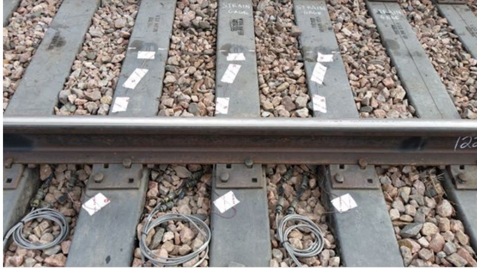
Figure 8. Instrumentation setup on the EPC ties
