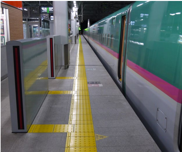
Figure 3-8. Examples of platform screen doors and barriers. Top: full-height doors in China [11]. Bottom-left: part-height solid barriers in Japan [29]; Bottom-right: barrier fences in Germany [13]
