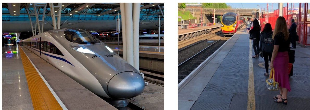
Figure 3-7. Examples of platform edge safety markings (left image [84])
