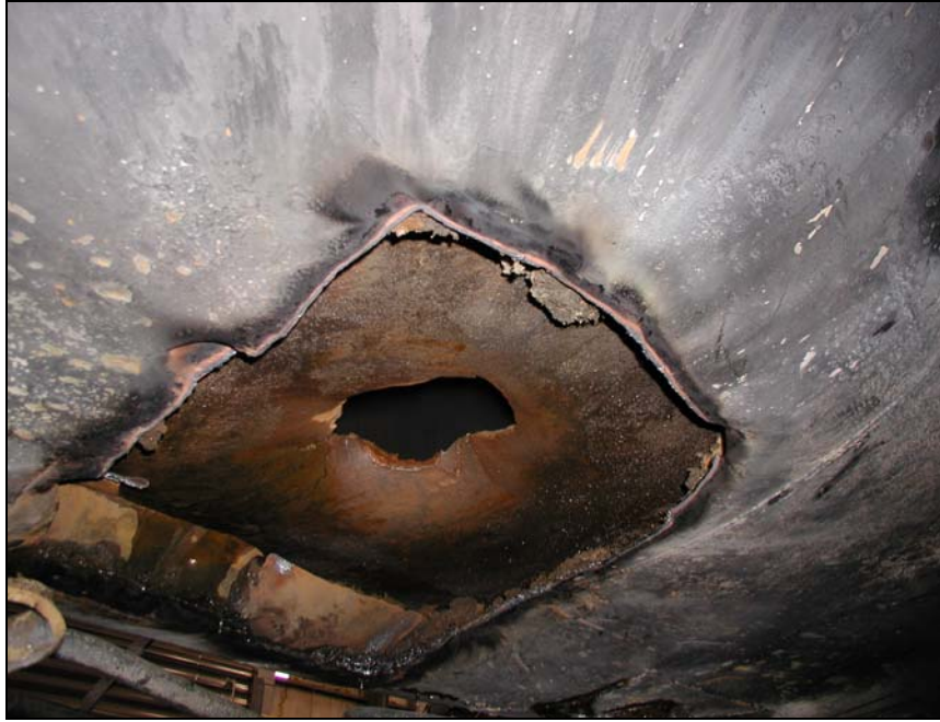
Figure 17. Drain Hole from Test 1 Using Helix-Shape Charge
