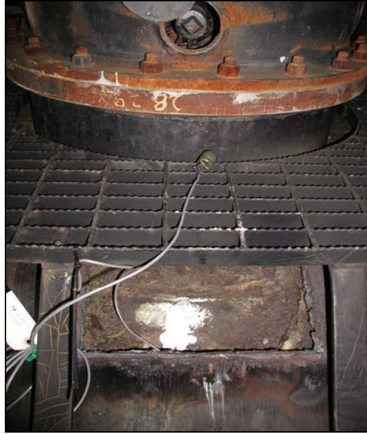
Figure 8. Strain Gage at Base of Manway
