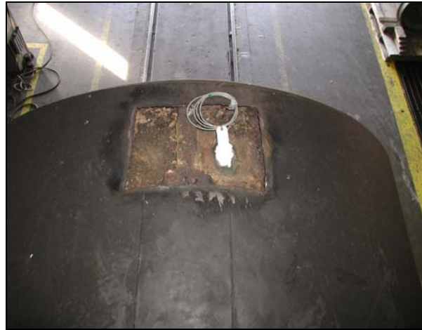
Figure 7. Strain Gage Near Shell to Head Weld, A-End
