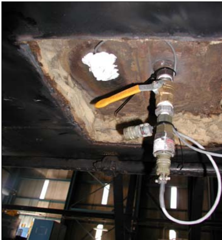
Figure 6. Pressure Transducer and Strain Gage on Bottom Surface of Tank
