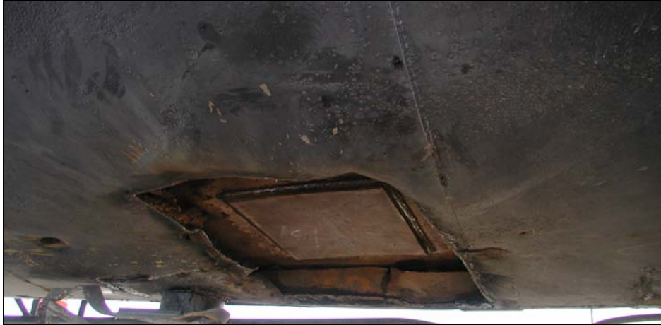
Figure 15. Patch Welded Over Drain Hole from Test 1
