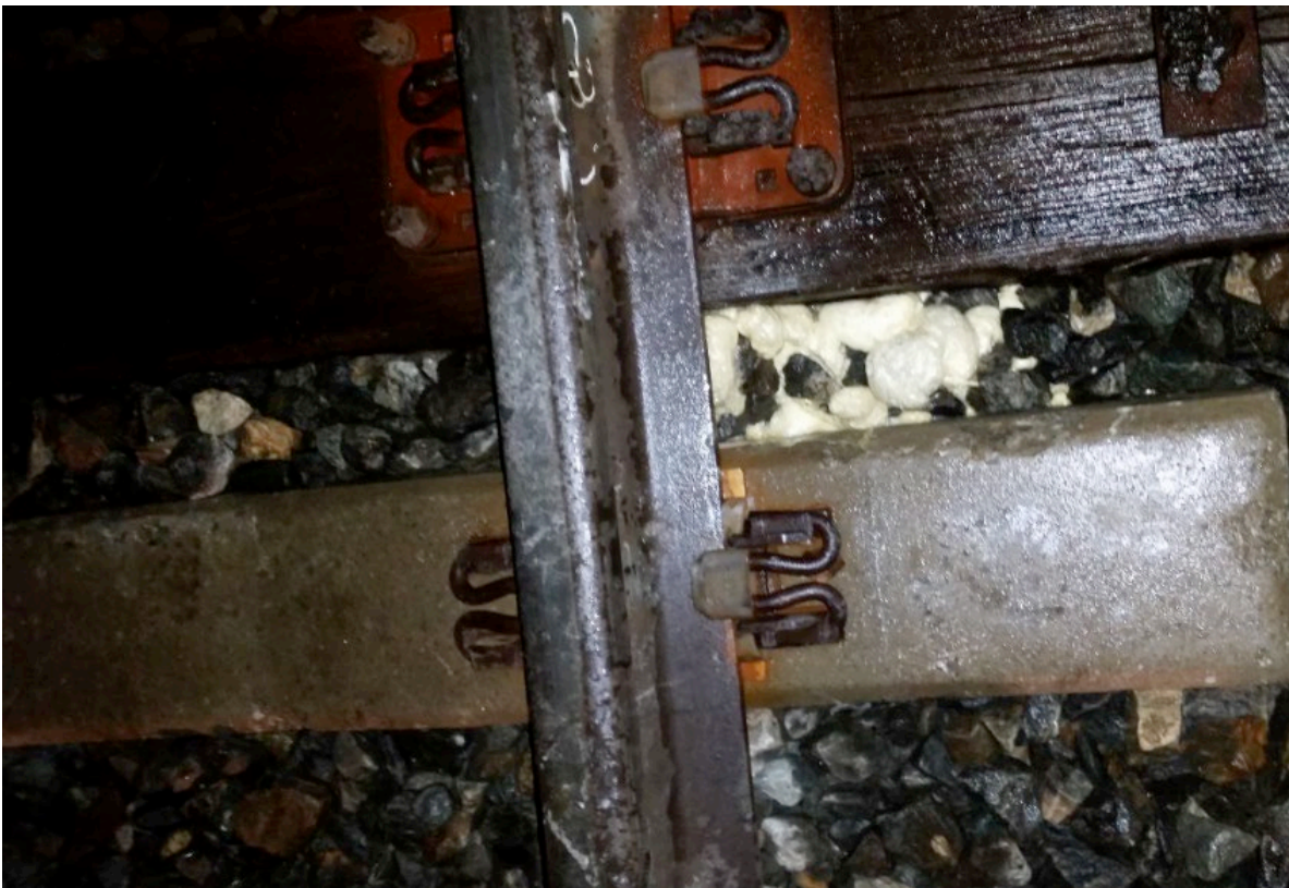
Figure 2.7: Polyurethane Grouting of Ballast – Injected Grout Seen From Underneath Tie
