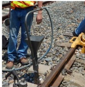
Figure 6.23: Different Steps Involved in the Stone-blowing Process
