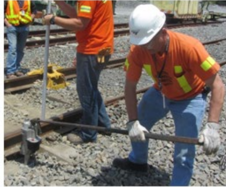
Jacking of Track to Pre-Determined Level
