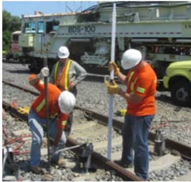
Surveying of Track to Establish Top-of-Rail Profile
