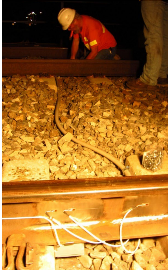
Figure 3.27: Installing Cable Duct Underneath Adjacent Tracks
