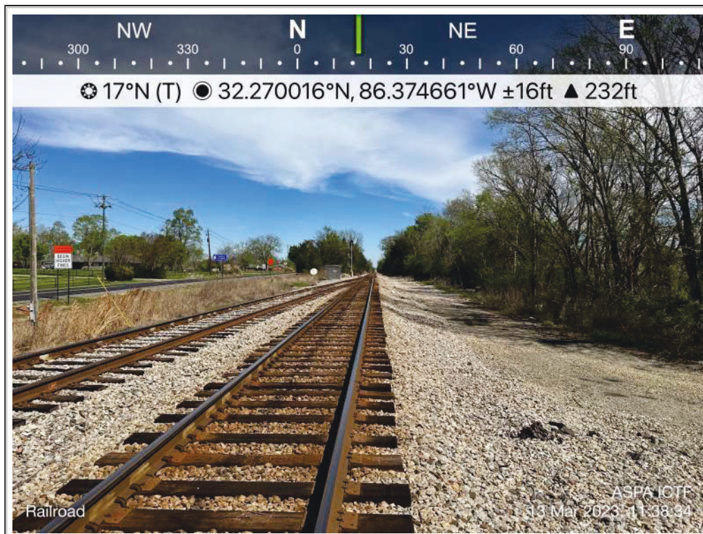
Picture 10: View looking north of railroad tracks at Wasden Road
