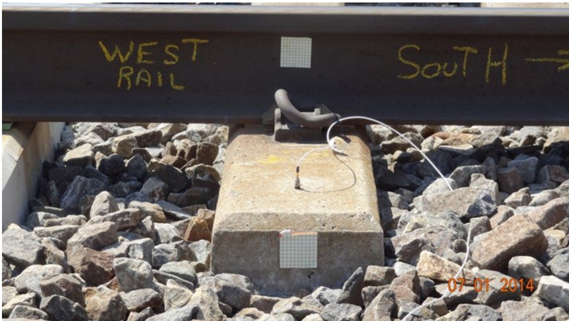
Figure 106. Accelerometer attached to concrete tie
