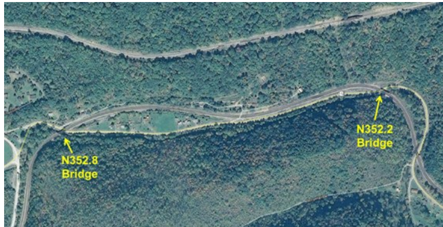
Figure 2. Aerial view of NS instrumentation locations near Bluefield, WV
