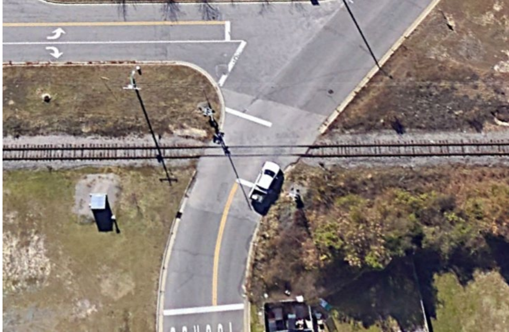
Figure 33: Satellite imagery showing crossing 847210G
