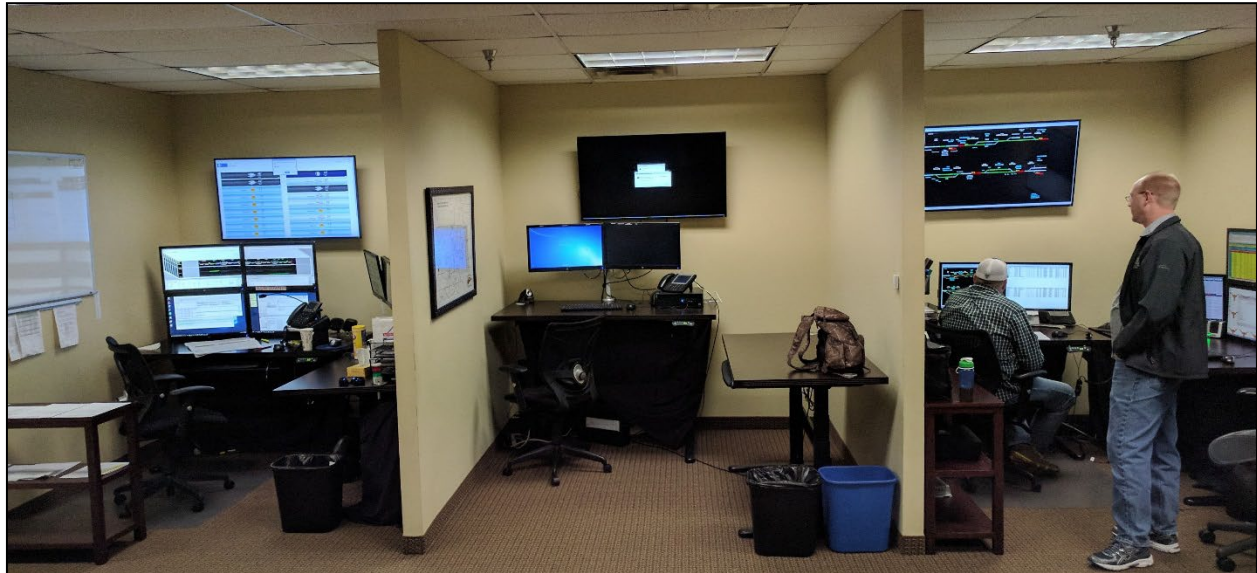
Figure 2. Rio Grande Pacific Company's Two Dispatcher Desks (left: shortline freight; right: local commuter)
