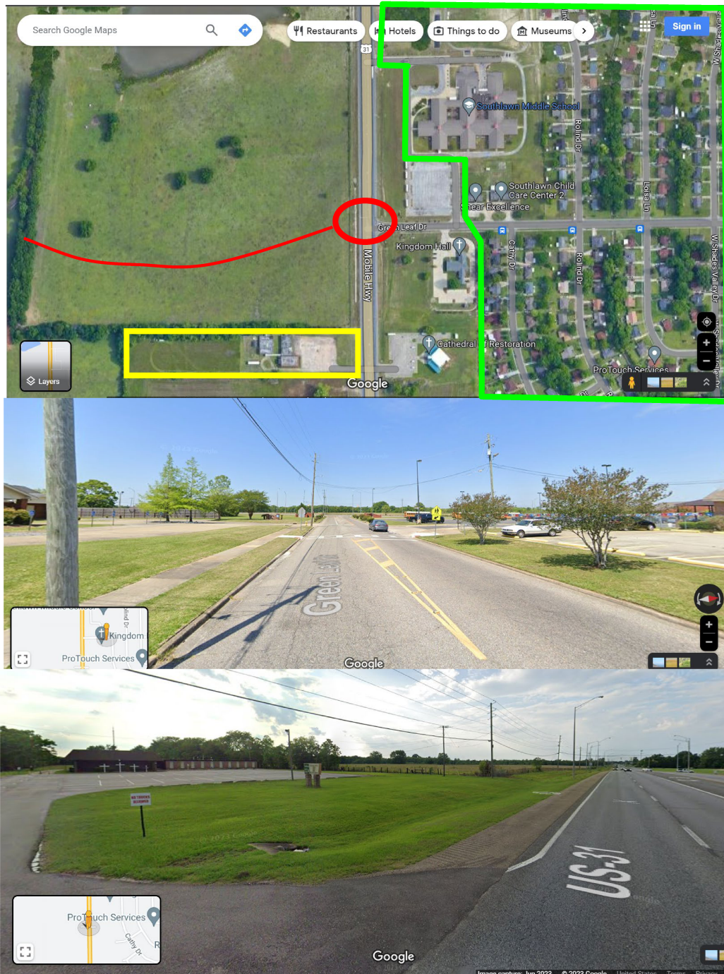
Figure 1. 2023 Google aerial view of Project area (top) with boundaries of the Southlawn Baptist Church in yellow and of the English Village and Southlawn Historic District (green), to which the church also contributes. The red circle shows the location of the intersection improvements, and the red line approximates the proposed new road (Attachment A for site plan). The middle image is from the edge of the historic district looking west to the intersection of Green Leaf Drive and US 31. The bottom image shows the entrance of the Southlawn Baptist Church looking north to the location of the intersection improvements.
