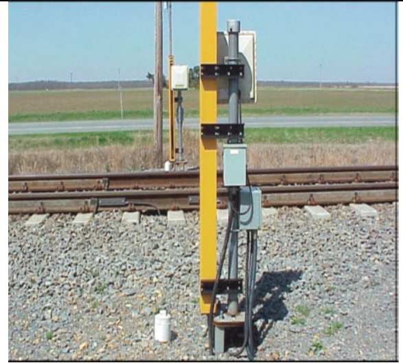
Figure 11: A Typical Low Air-Hose Detector
