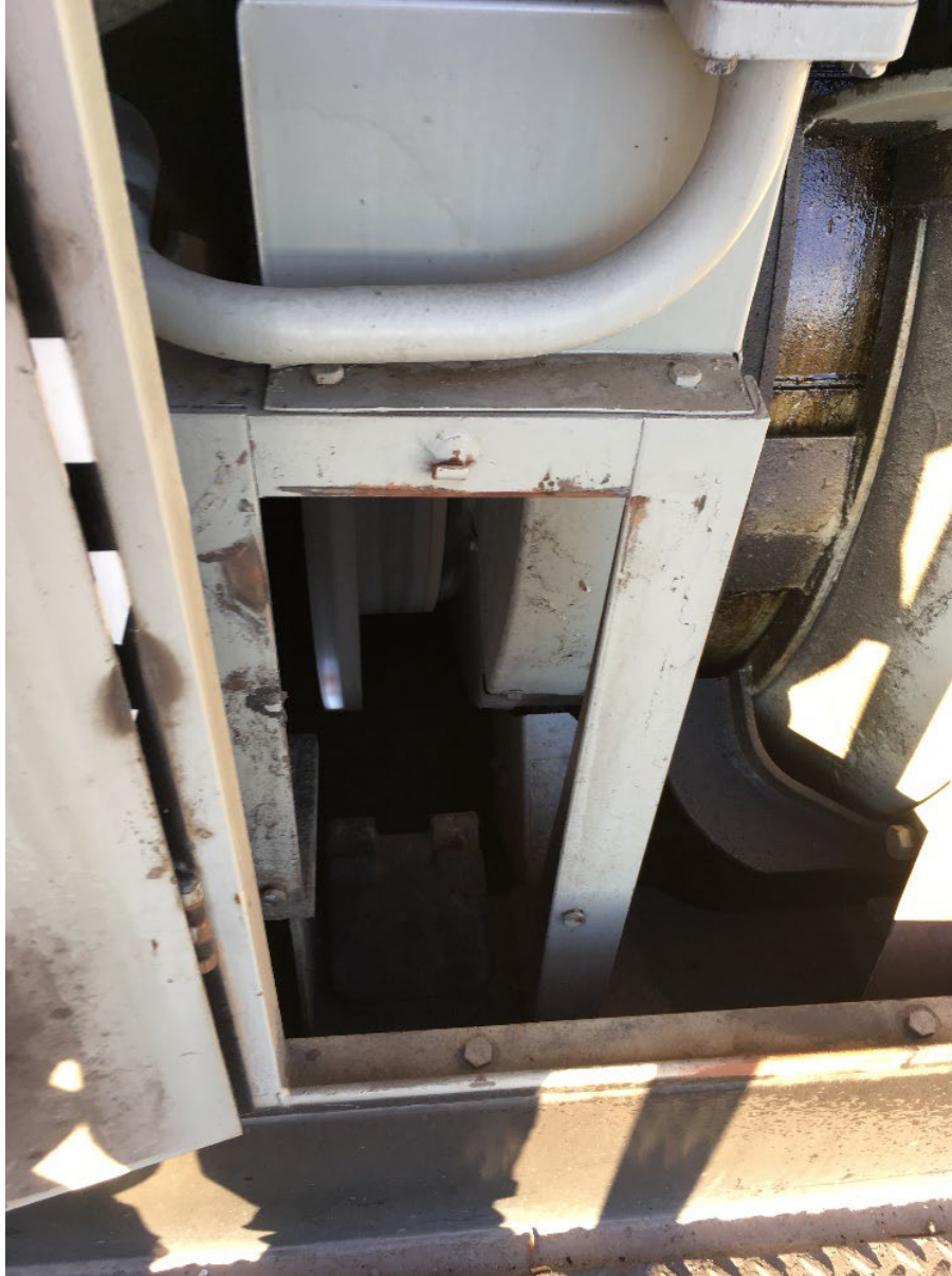
Figure 2: Missing flywheel cover on EMD locomotive.
