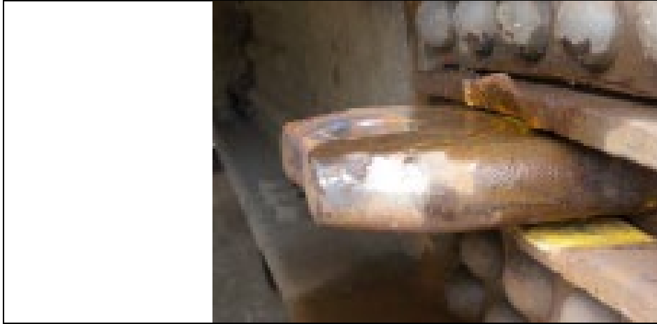
Missing retainer
