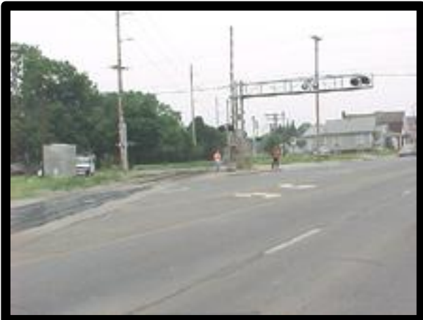
Figure 3. Southeast corner facing northeast.
