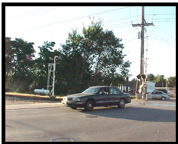
Figure 6. Southeast corner facing northwest.
