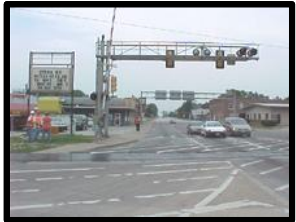
Figure 2. Southwest corner facing north.
