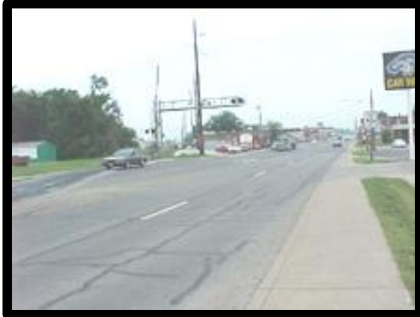
Figure 1. Northeast corner facing west.
