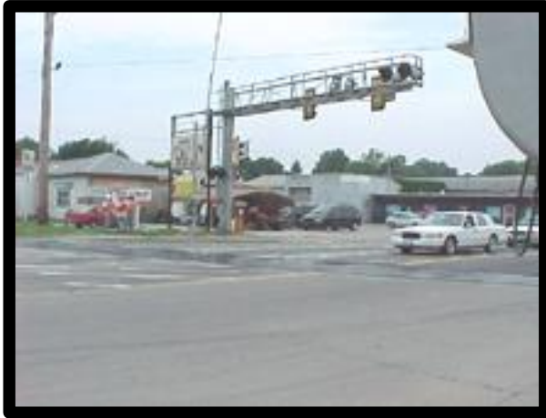
Figure 1. Southeast corner facing northwest.
