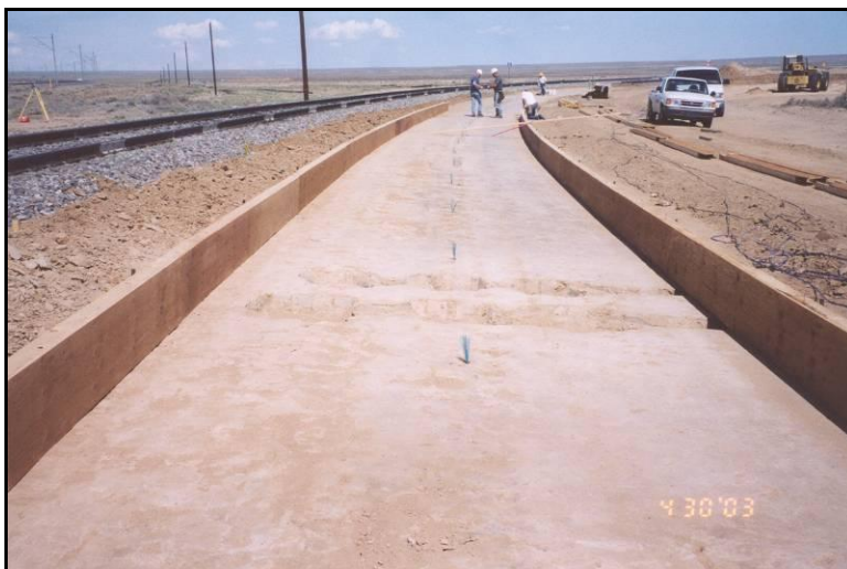
Figure 8. Soil Cement Subbase Surface for Slab Track Test Section
