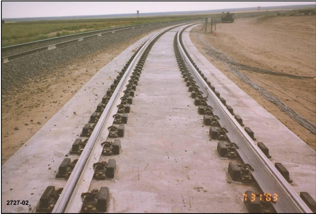
Figure 16. Views of IDBT (top) and DFST (bottom) following Construction
