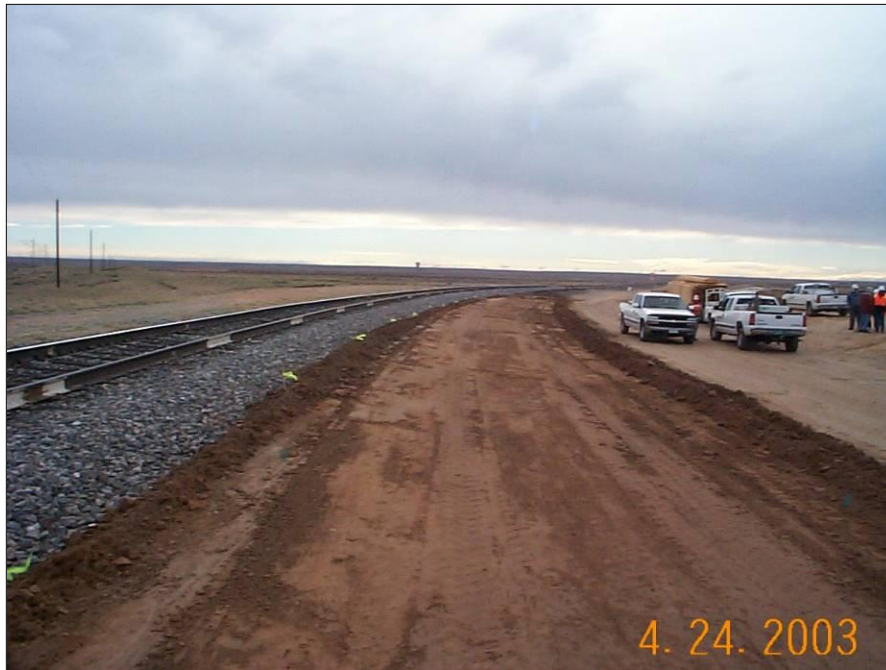
Figure 7. Subgrade Surface for Slab Track Test Section
