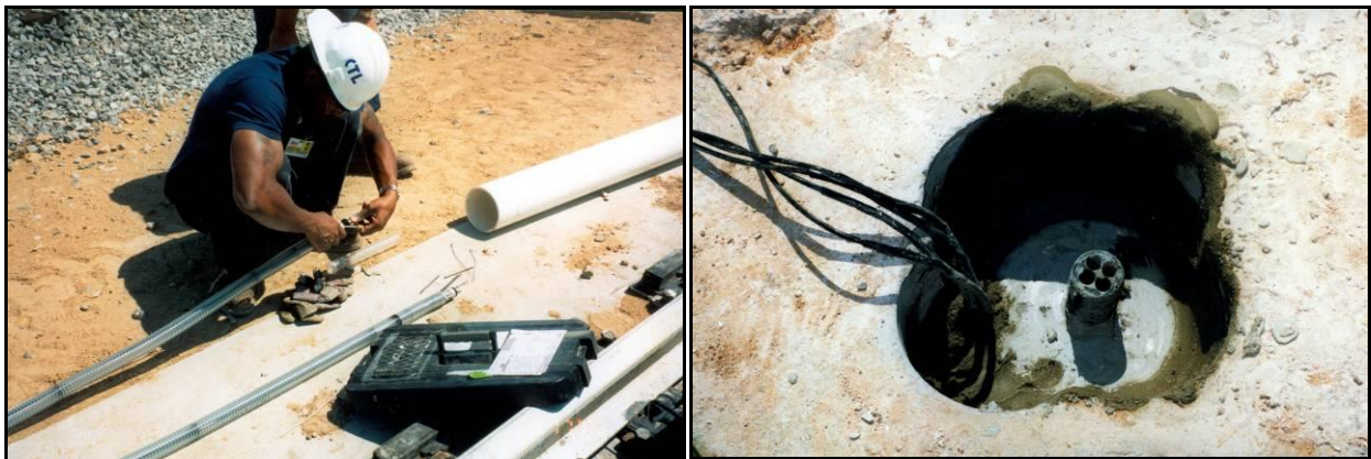
Figure 55. MDD before and after Installation in Slab Track
