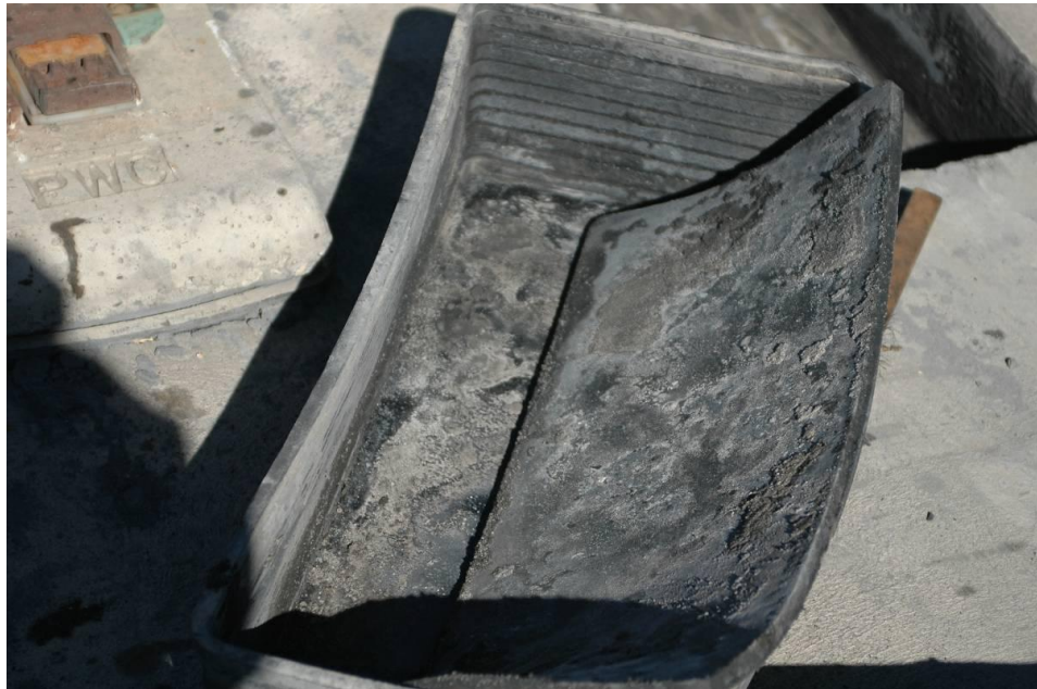
Figure A10. Pad of Tie Number 151
