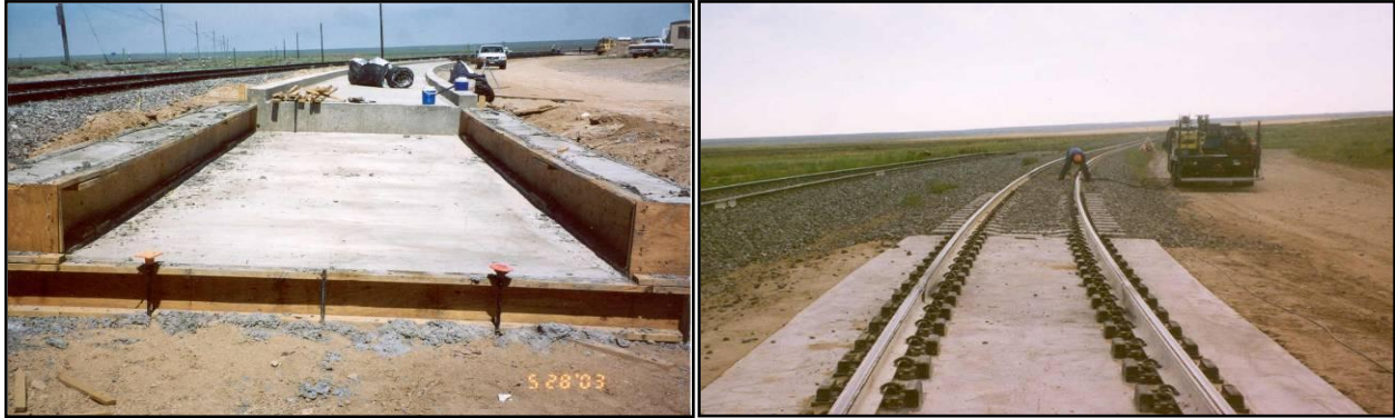
Figure 15. Base Slab in Transition to the IDBT and DFST Transition
