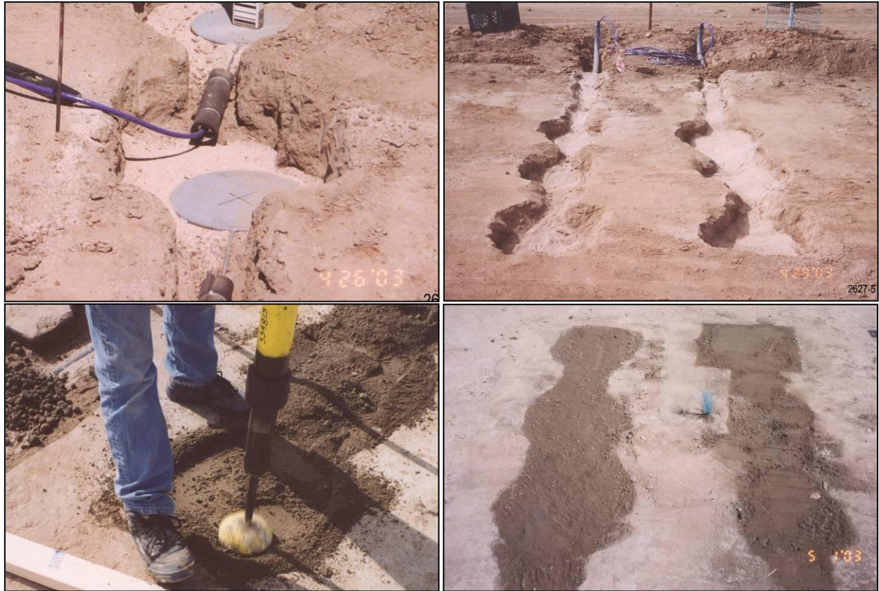
Figure 66. Installation of Subgrade Pressure Cells
