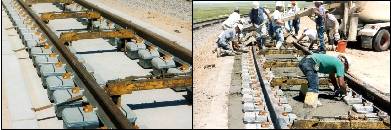
Figure 12. Construction of the IDBT Using Top-down Method
