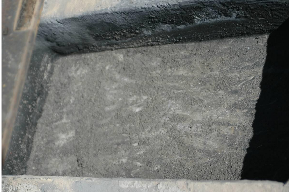
Figure A7. Cavity of Tie Number 151, Showing Sand in the Bottom
