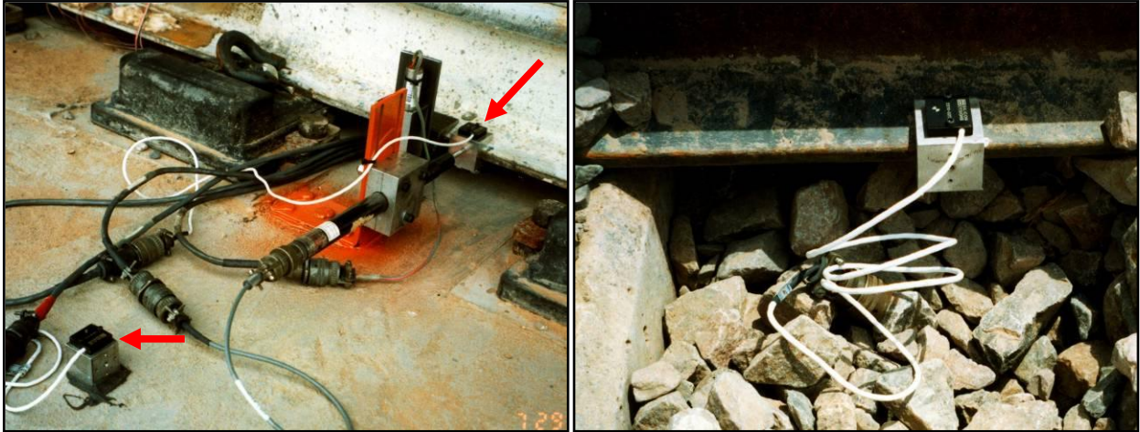
Figure 70. Accelerometers Installed in Slab Track (arrows) and in Transition
