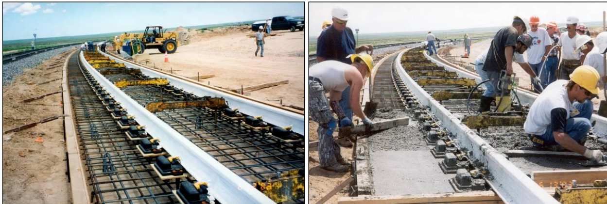
Figure 10. Construction of DFST Using Top-down Method
