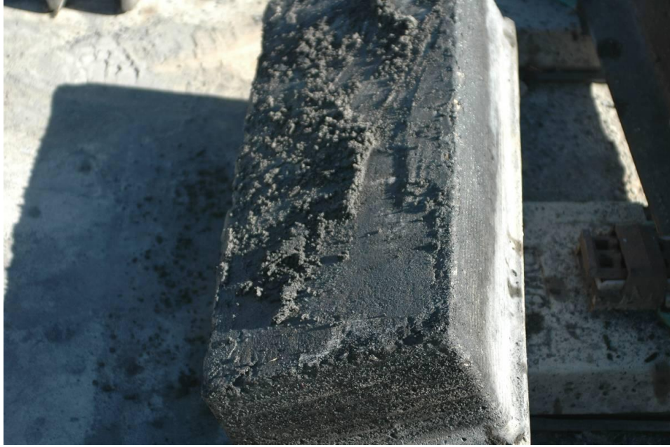
Figure A11. Bottom of Tie Number 152
