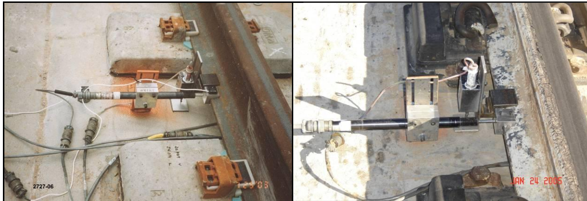
Figure 53. LVDT for Vertical and Lateral Rail-to-Slab Deflection (IDBT and DFST)
