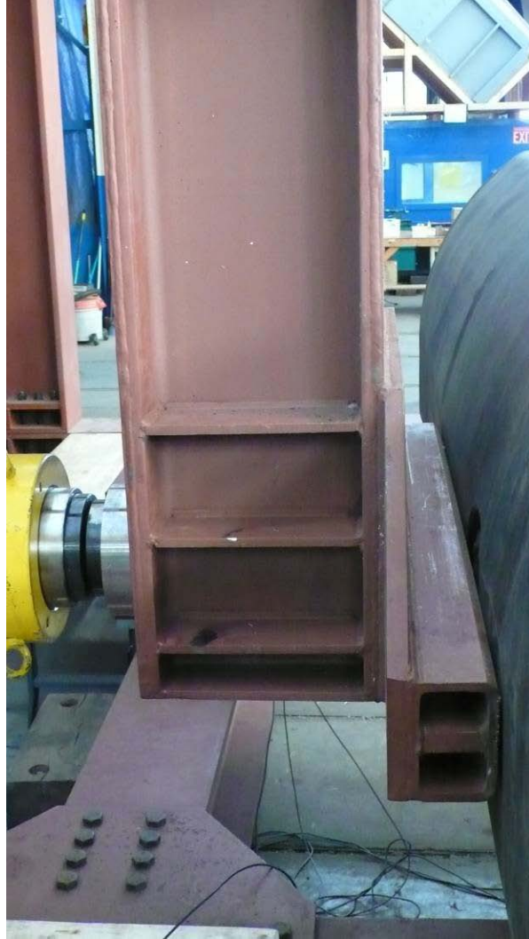
Figure 10. A Closeup View of Tank Sidewall and the Load Lever following Complete Unloading
