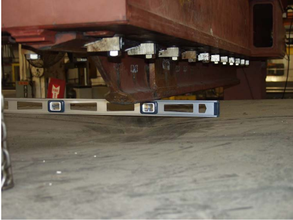
Figure 16. Posttest Closeup View of Deformed F59 Tank Bottom Wall
