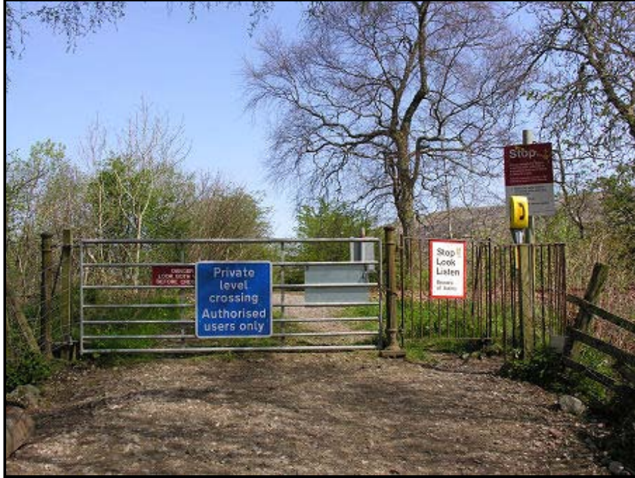
Figure 25. Private Highway-Rail Grade Crossing in Great Britain
