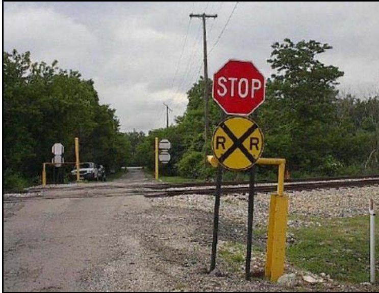
Figure 36. Additional Private Crossing Signage Example
