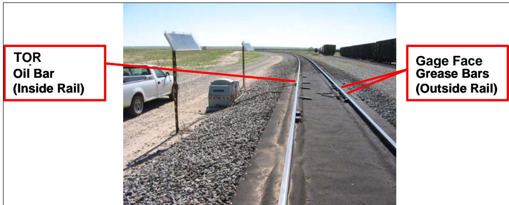
Figure 3. FAST Loop Lubrication Site in Section 24, with Gage Face Grease (High/Outside Rail) and TOR Oil (Low/Inside Rail) Applicator Bars Indicated
