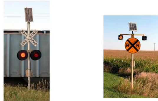
Figure 2. (left) Mn/DOT Flashing Lights with Solar Panel and (right) Advance Warning System [5]
