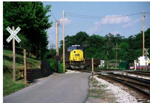
Figure 1. A Typical Passive Crossing (Secretary's Action Plan for Highway-Rail Crossing Safety and Trespass Prevention 1994)
