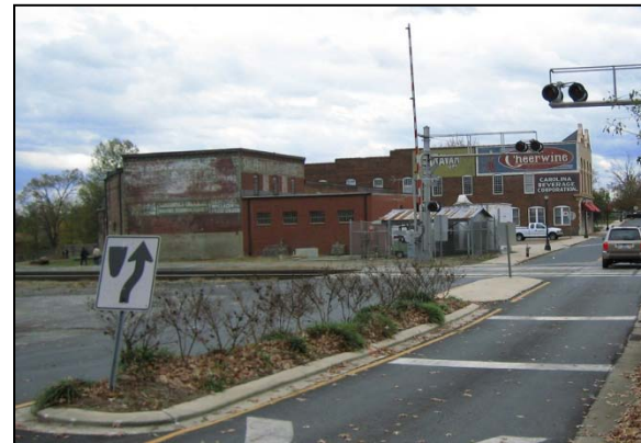
Figure 2: Wide Raised Median
