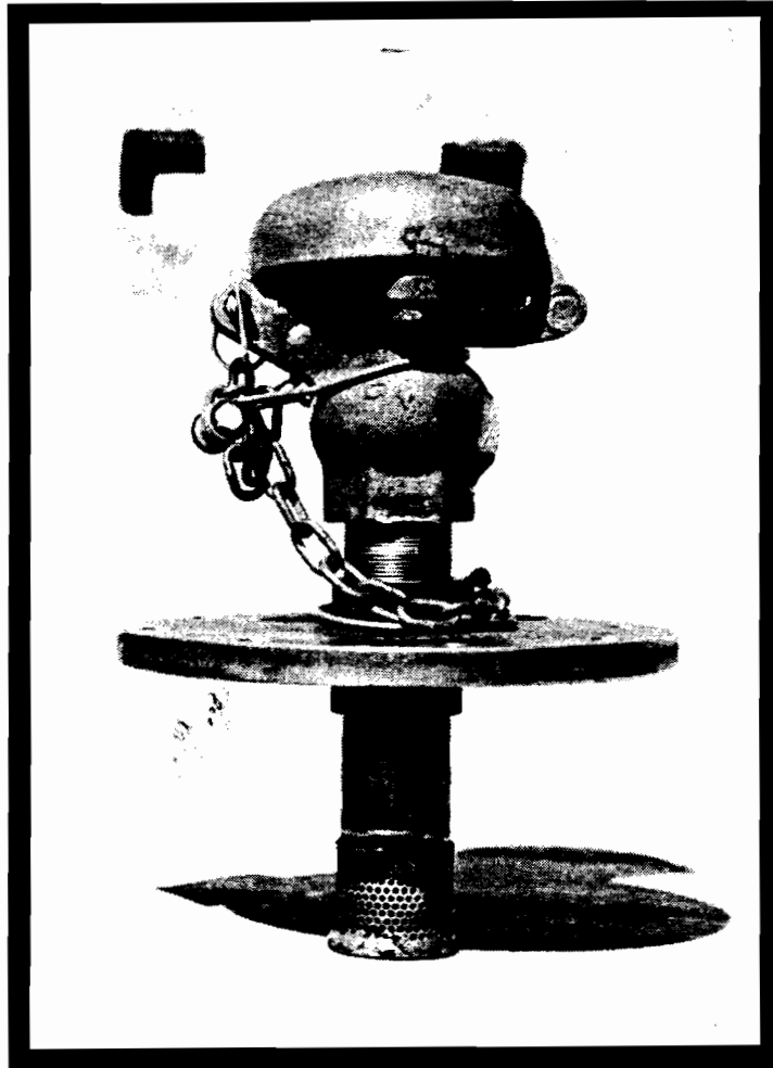
Figure 10. View of Safety Vent/Mesh Type SPR for 6 1/2" Safety Vent
