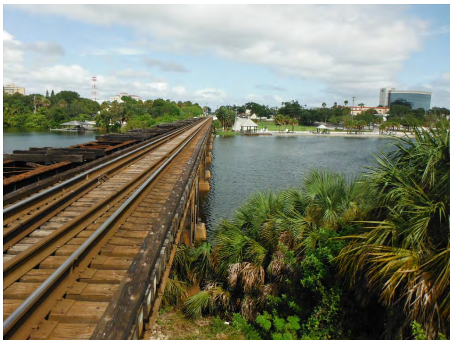
Photograph 4. Crane Creek Bridge (Mile Post: 194.47), Facing north toward to the waterside park
