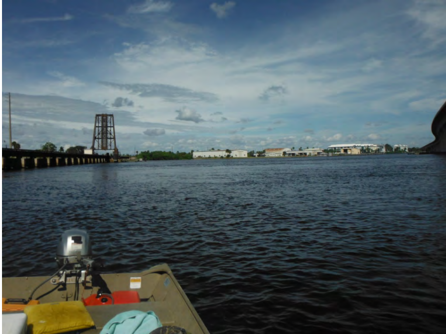
Photograph 10. St. Lucie River Bridge (Mile Post 260.93), Facing north across the St. Lucie River
