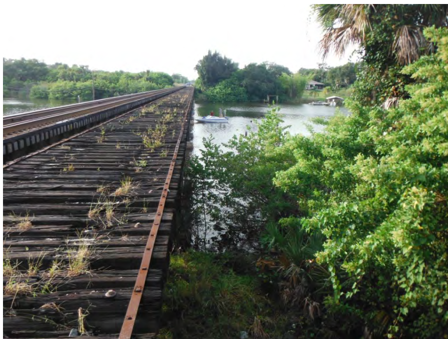
Photograph 1. Eau Gallie River (Mile Post: 190.47), Facing south across the Eau Gallie River
