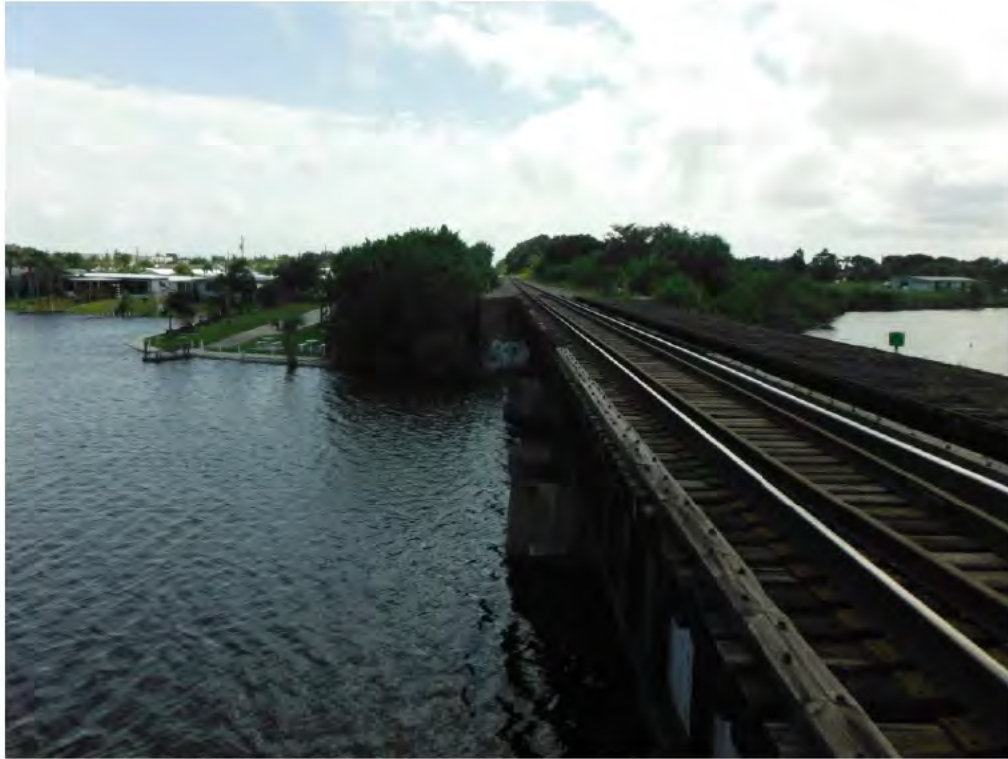
Photograph 5. Turkey Creek Bridge (Mile Post 170.70), View facing north.
