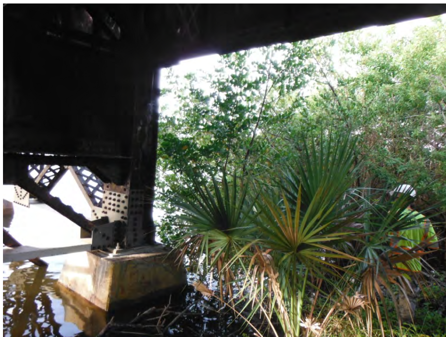
Photograph 2. Eau Gallie River (Mile Post: 190.47), White mangrove and saw palmetto growing beneath the bridge
