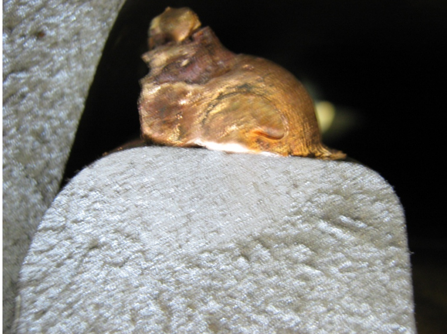
Figure 48. CAD Weld Driven Failure due to Formation of Martensite
