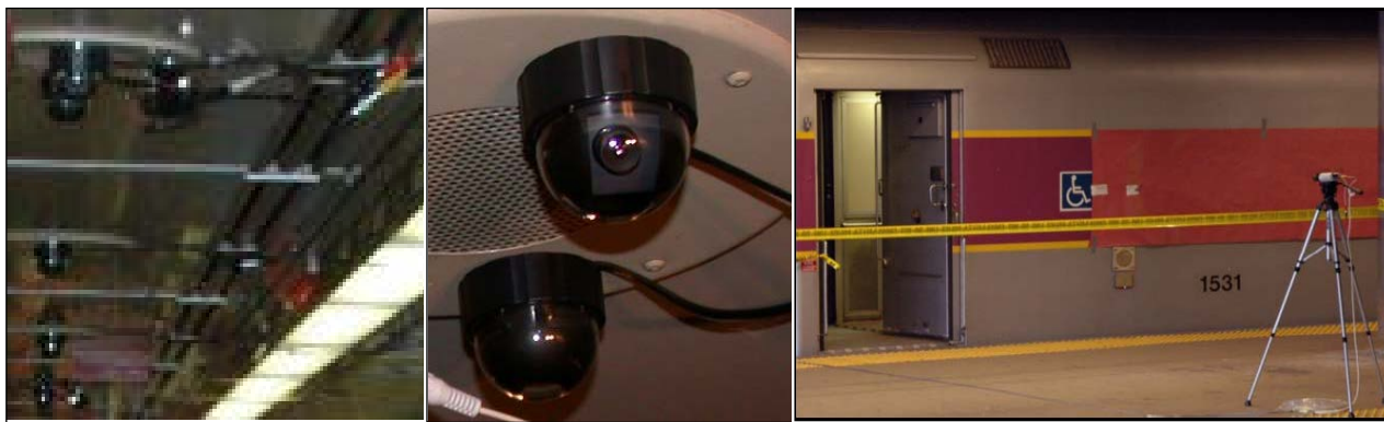
(a) Interior Ceiling
