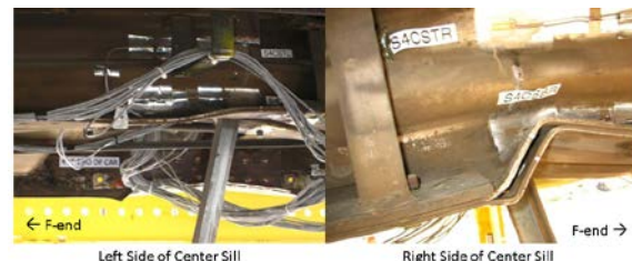
Figure 6. Buckle on the Center Sill
