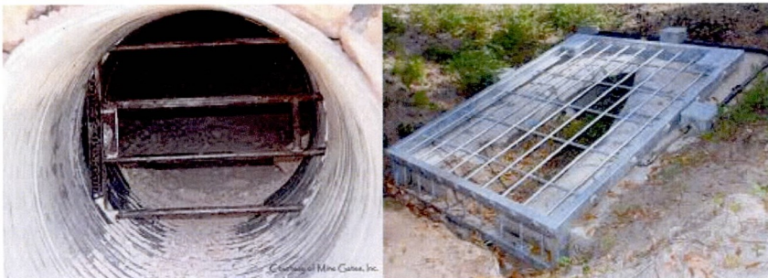
Figure 2. Examples of a traditional culvert gate (left) and angled culvert gate (right)
