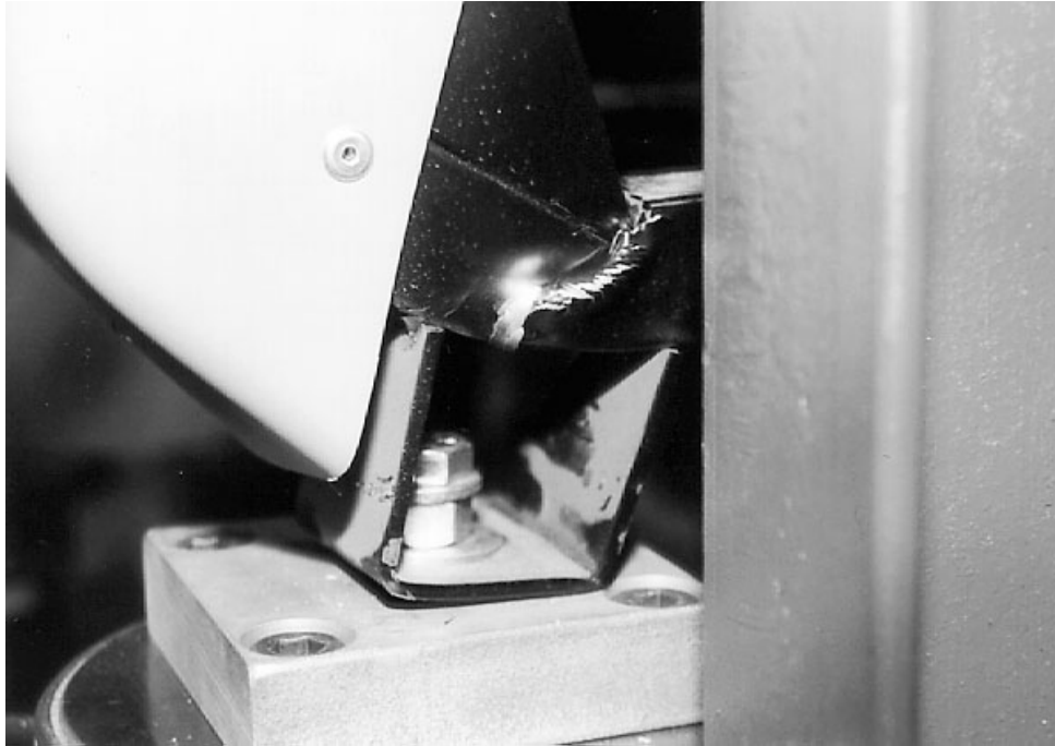
Figure 15. M-Style Upper (Post-test) - Square Beam Attachment Buckled
