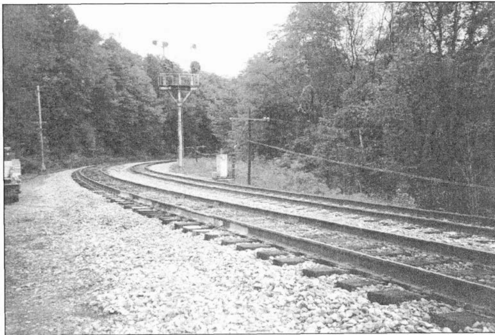
Figure 5. WV Monitoring Station Site at MP 251.7
