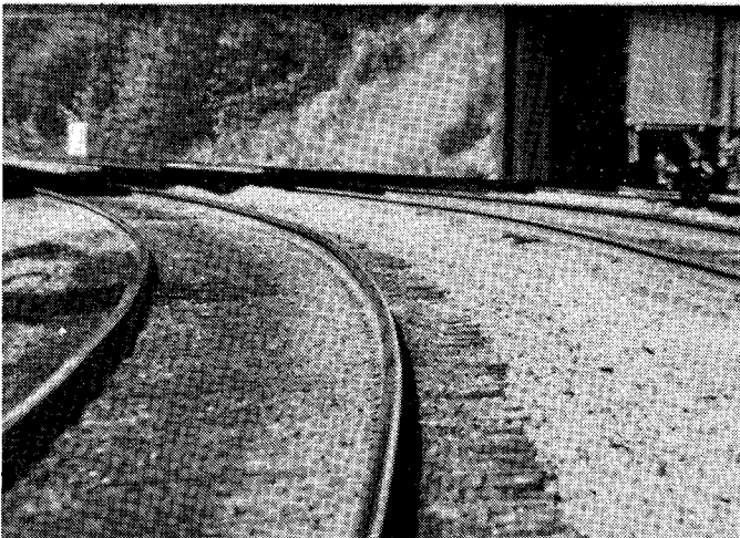
(c) Alignment Kinks in Spiral, Location C, Looking West
