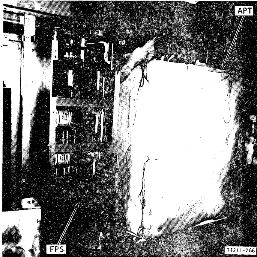
b. INSTALLED IN MOCKUP, FPS COVER AND AUXILIARY POWER TRANSFORMER ENCLOSURE PANELS REMOVED
