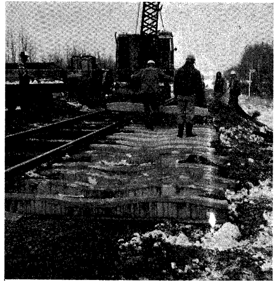
Ties Prior to Installation Fig. E-2
