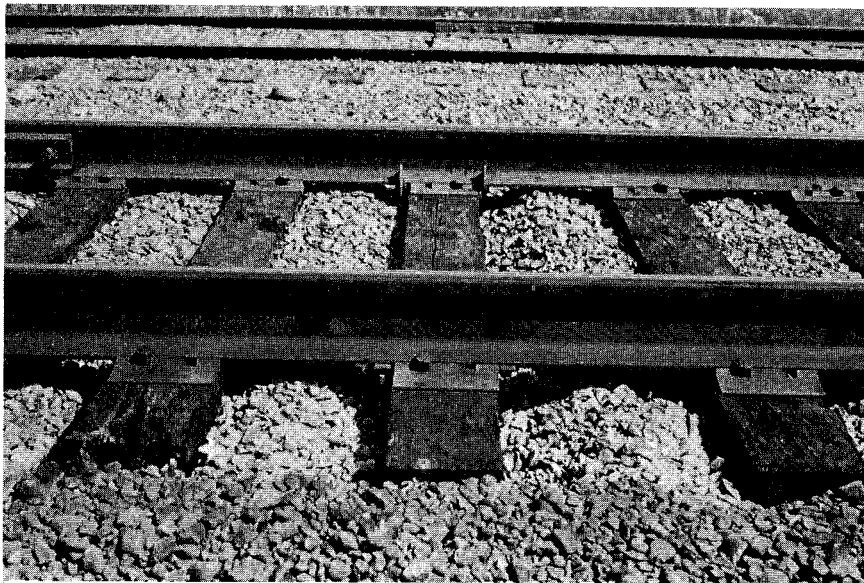
First Sign of Back and Forth Tie Movement - July 1974 Fig. F-6
