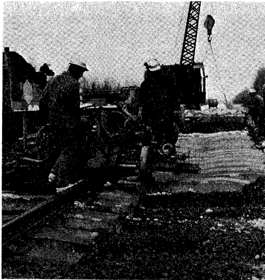
Installation of Ties Fig. E-3
