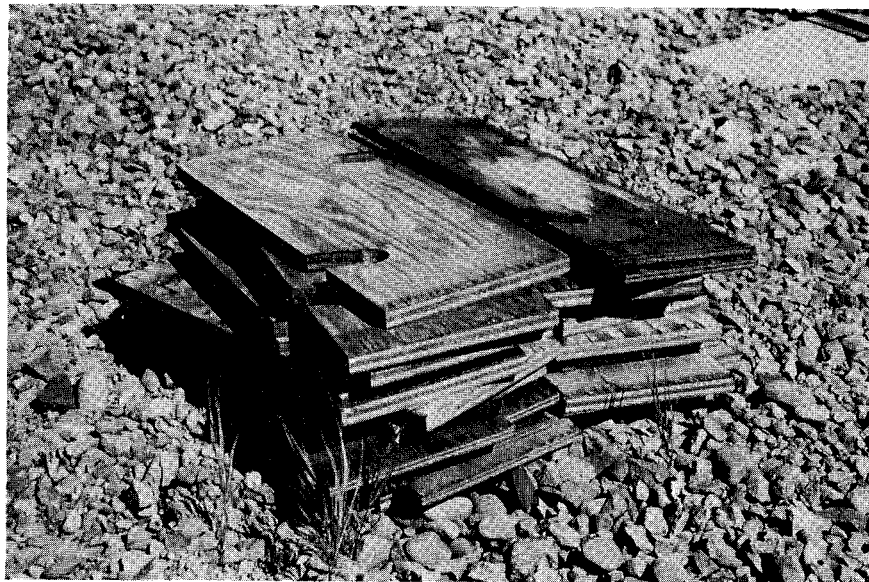
Wood Shims Removed After First Winter Fig. E-8
