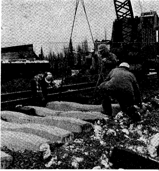
Positioning of Ties Fig. E-1
