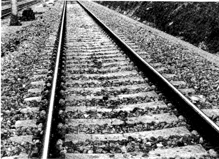
FIGURE 12. TEST ZONE IN MONOBLOCK CROSSTIE TRACK
