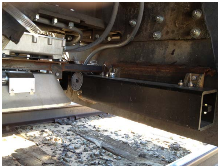
Figure 3. Transponder Scanner and Track Receiver
