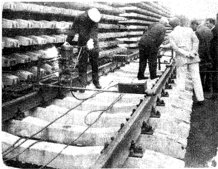
Figure 41. Tightening of Rail Fasteners
