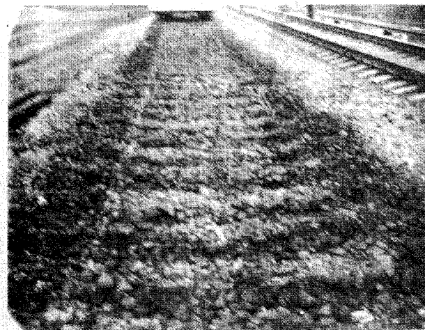
Figure 24. Ballast Under Removed Panel
