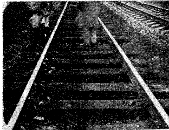
Figure 30. Ballast Behind SCHOM-DO Ballast Cleaner
