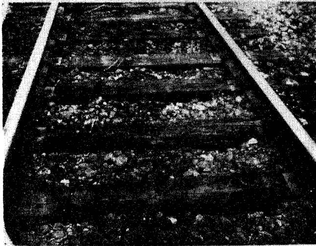
Figure 29. Condition of Ballast and Track Prior to Heavy Rebuild
