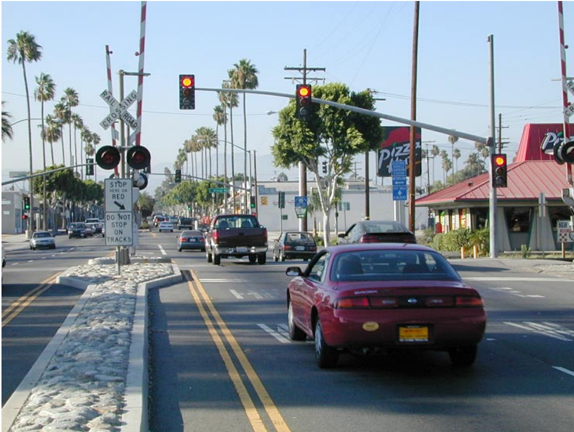
Figure 52. Pre-Signal with Louvered Downstream Intersection Signal, Sierra and Orange at Metrolink Commuter Line, Fontana, California
