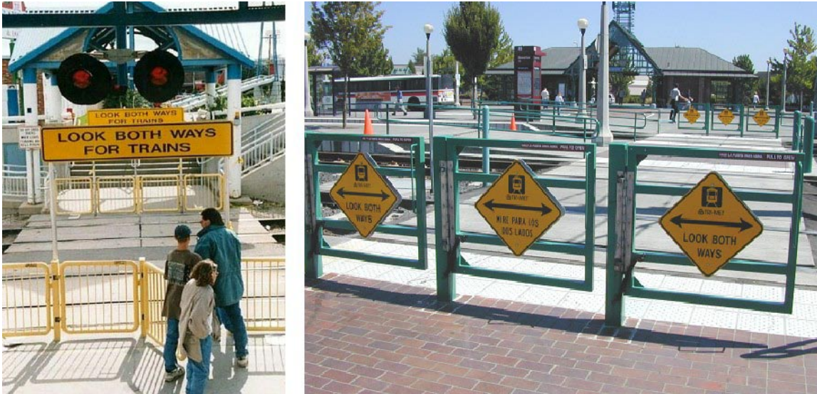
Figure 77. Pedestrian Swing Gate Examples
