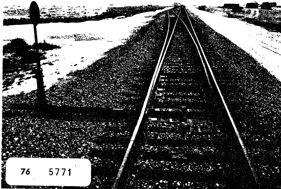
FIGURE 10. WEST BY-PASS TURNOUT LOOKING CCW.
