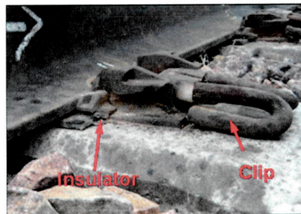
Figure 1: Example of Rail Fastener for Concrete Tie Track (Note-note that the clip shown is not engaged on the rail)
