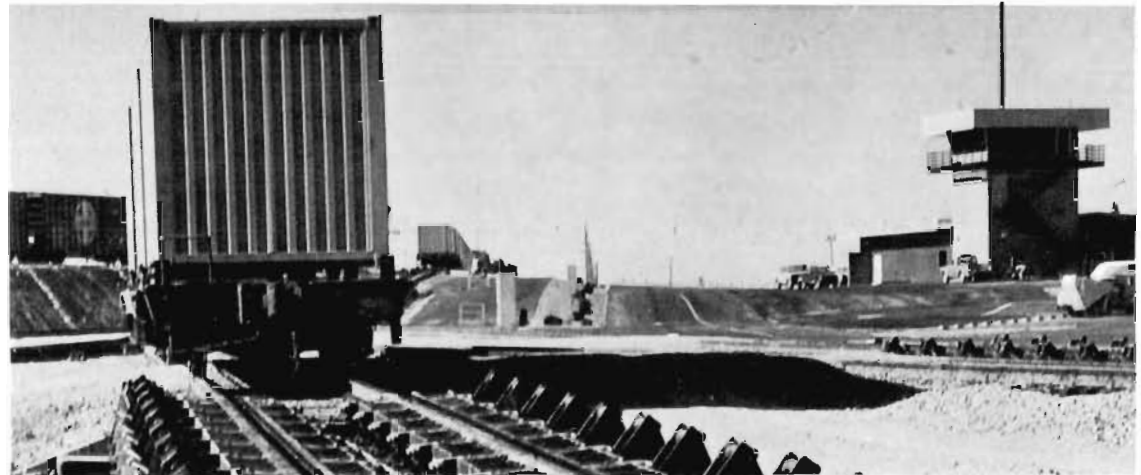
CONVENTIONAL CLASP-TYPE CAR RETARDER SYSTEM
