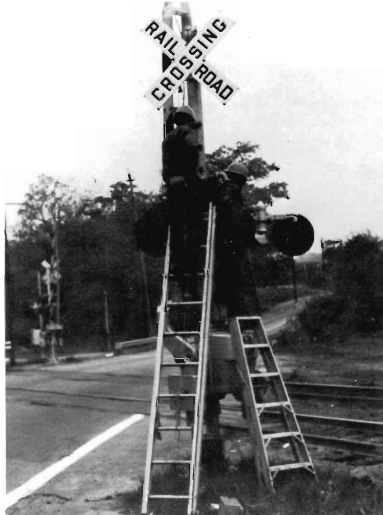
IMPROVEMENTS BEING MADE AT A RAIL-HIGHWAY GRADE CROSSING
