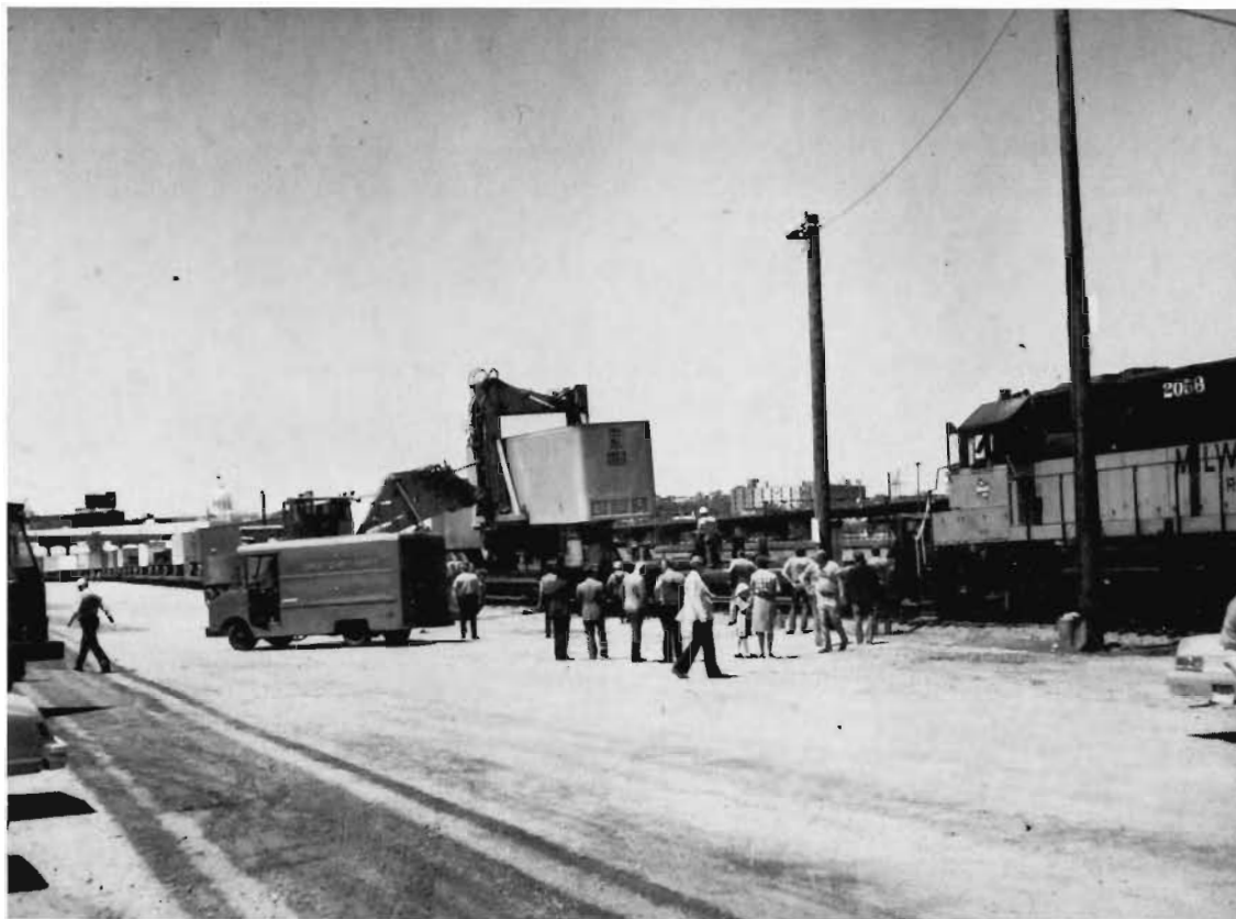
LOADING TRAILERS ON BOARD A SPRINT TRAIN ON THE FIRST DAY OF SERVICE
