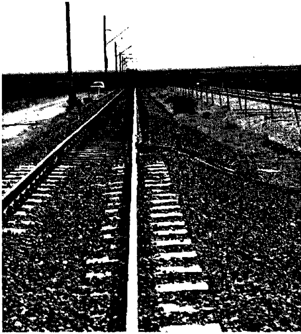
1) TANGENT TRACK WITH STIFFENED ENDS
