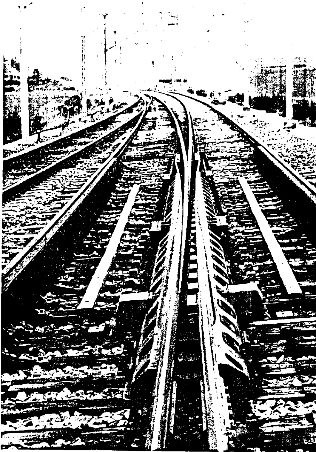
Figure II.1.5 Moveable Frog Turnout on LGV-PSE
