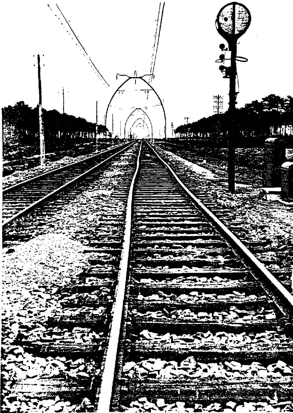
Figure II.1.2 Track Condition After the French 205 MPH Record Runs in 1955
